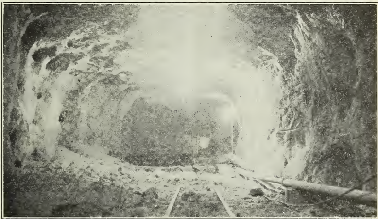
FIGURE 4.—Typical drift in potash mine, Carlsbad, N. Mex. Entire tunnel is through potash ore. Holes in left side are experimental borings with mechanical auger
